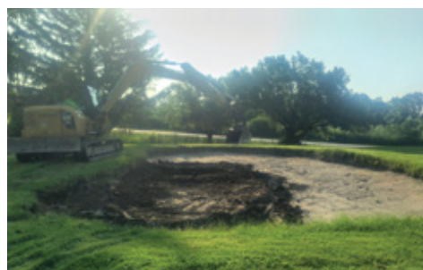
Sand trap on hole #9: Before, during excavation, and finally being filled with new sand.
